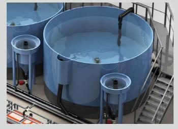
Particle separator and tank with double discharge through which 85 % of the water passes out through an auxiliary discharge and is brought to the discharge pipe. The remaining water is discharged through a centre discharge pipe in the bottom and must pass the particle separator before it is transported to the discharge pipe and cleaning in a mechanical
